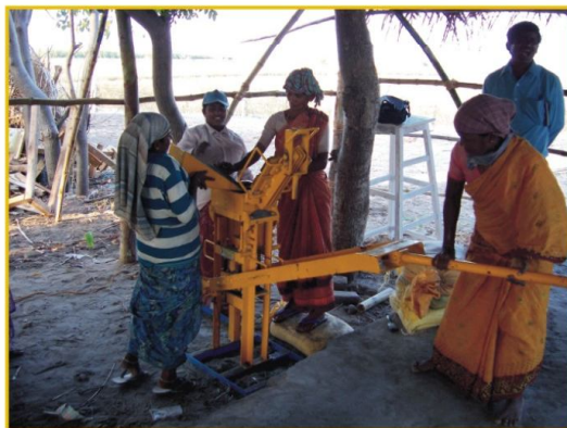
TARA Balram in operation
